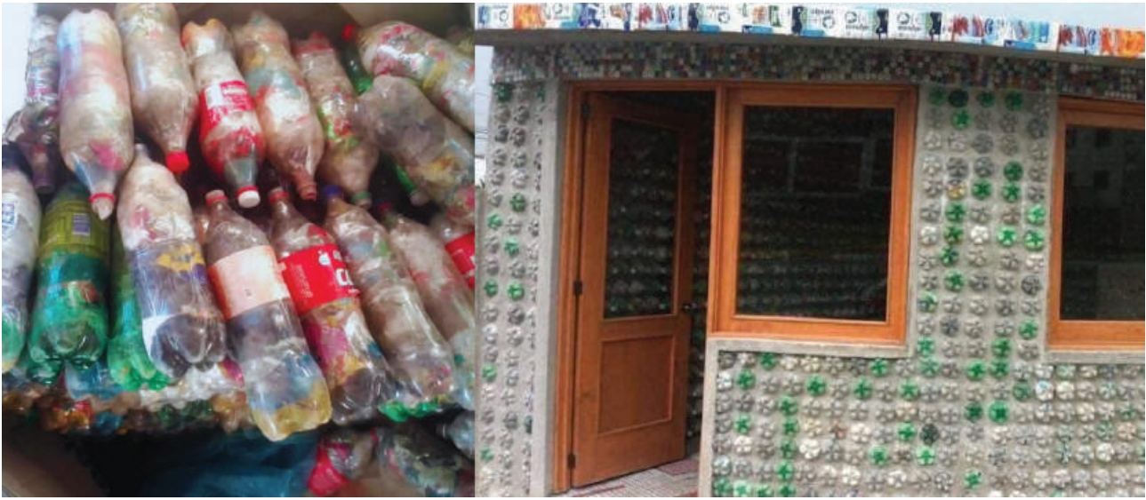
Iloilo City showcase an ECO Brick, a project of St. Therese MTC Colleges to build housing units using ECO Bricks.
