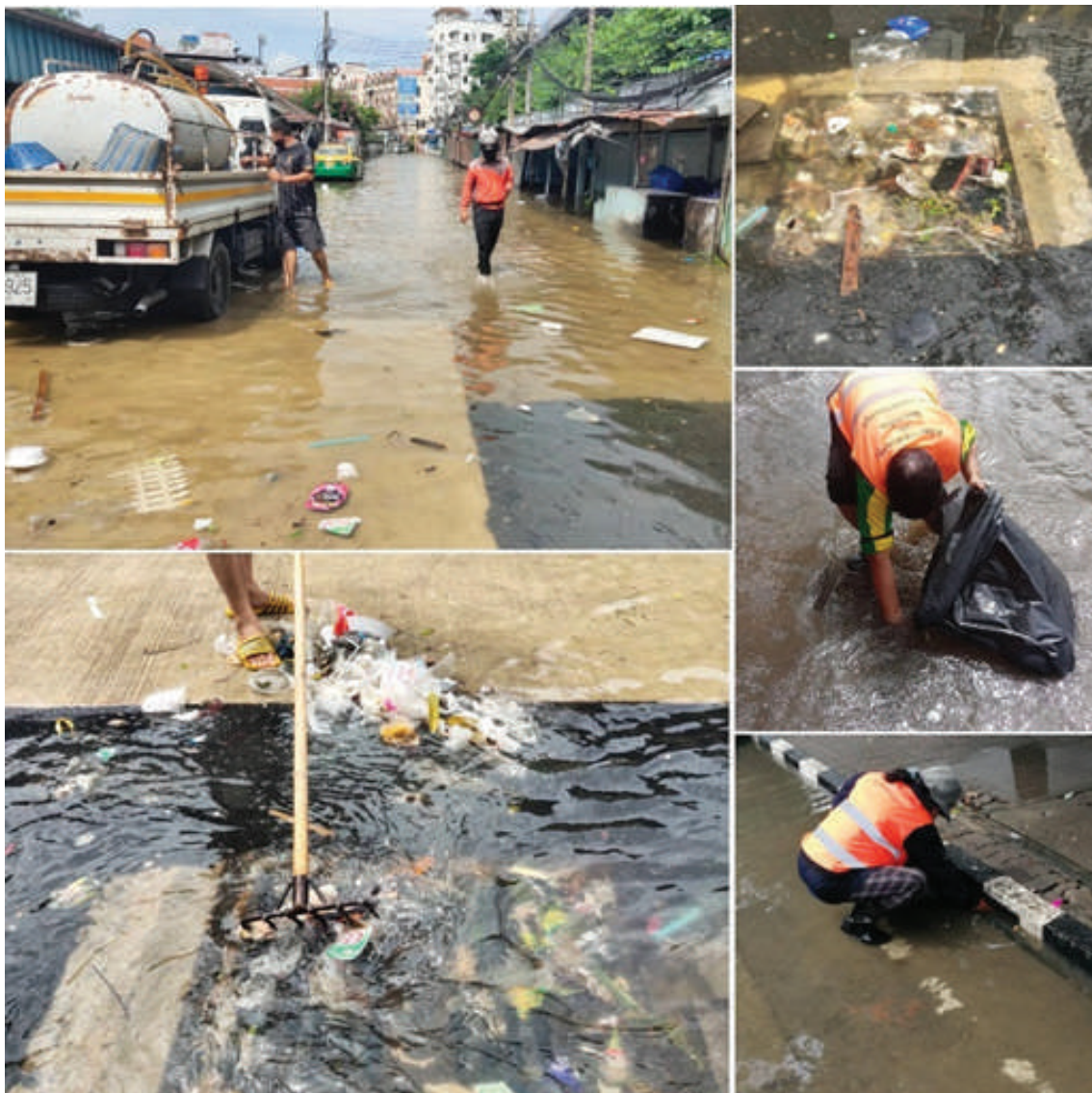
Figure 17. The waste clogged up the Drain in Nonthaburi municipality
