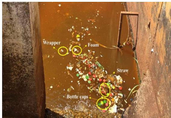
Figure 9.2. Trapped Plastics in the Preliminary Screening Process of a Wastewater Treatment Plant in the Lao PDR
